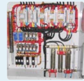
Close Transition Star-delta Starter
