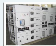
Factory assembling of L. V. Switchboard(s)
